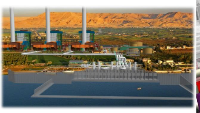
The power block is comprised of three identical Rankine cycle turbine generator units, each with a nominal rated capacity of 650 MW. The units are capable of generating rated capacity using natural gas, residual (mazout) oil, or a combination of both.
