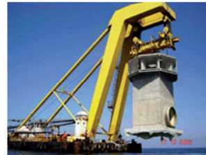
Intake Head Offshore structure
